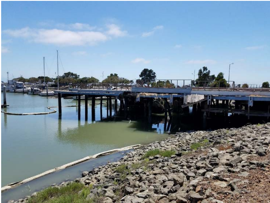
Photo 9 - Blue Dolphin Restaurant Foundation
