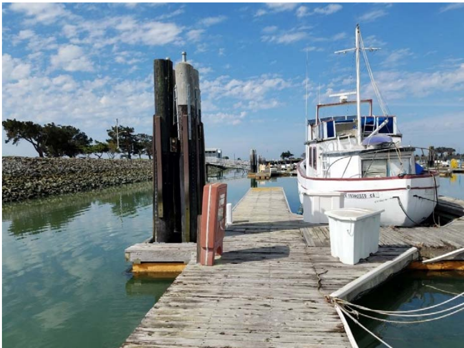
Photo 4 - Typical timber dolphin and floating dock. Note fiberglass jacket and concrete cap on the piles.
