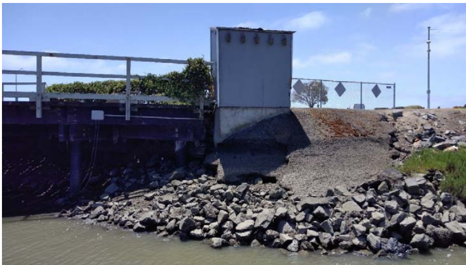
Photo 14 - Plywood Shed and Pile-Supported Closed Observation Deck
