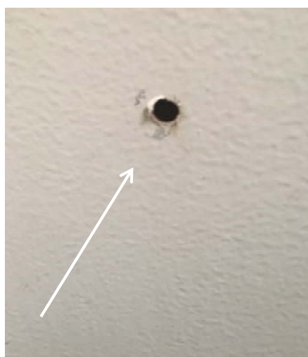
Photograph 2 – Marina – Restroom E, F – Wall texture (white) – Sampled at wall systems (indicated by white arrow) reported to contain asbestos.
