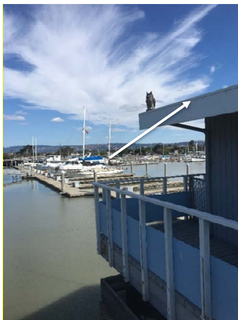
Photograph 7 – Marina – Harbor Master's Office – Flashing and sealant (grey) (typical, indicated by white arrow) and reported contain asbestos.
