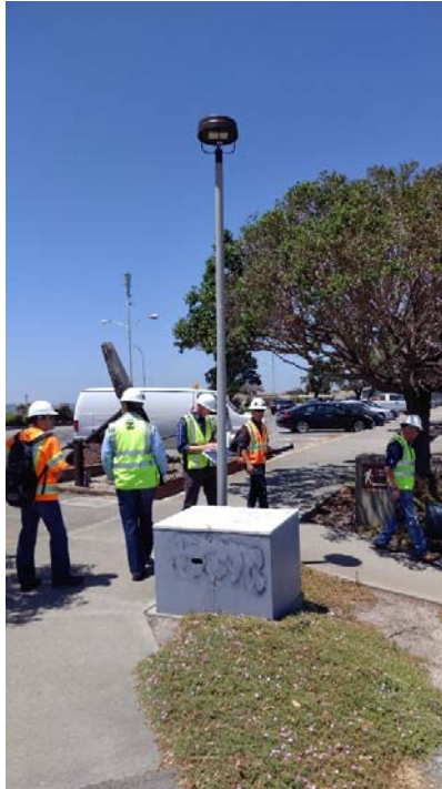
Photo 13 - Butane Tank Cabinet
