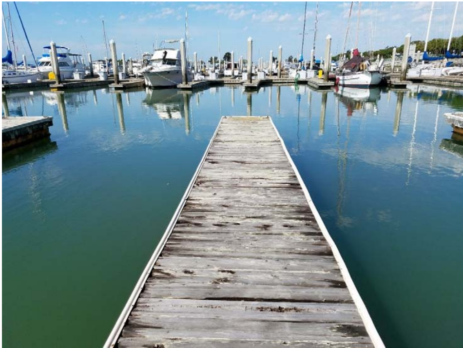
Photo 3 - Typical Condition of Timber Finger
